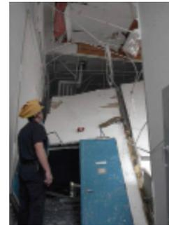
*Damage from Hydrogen Build Up*
